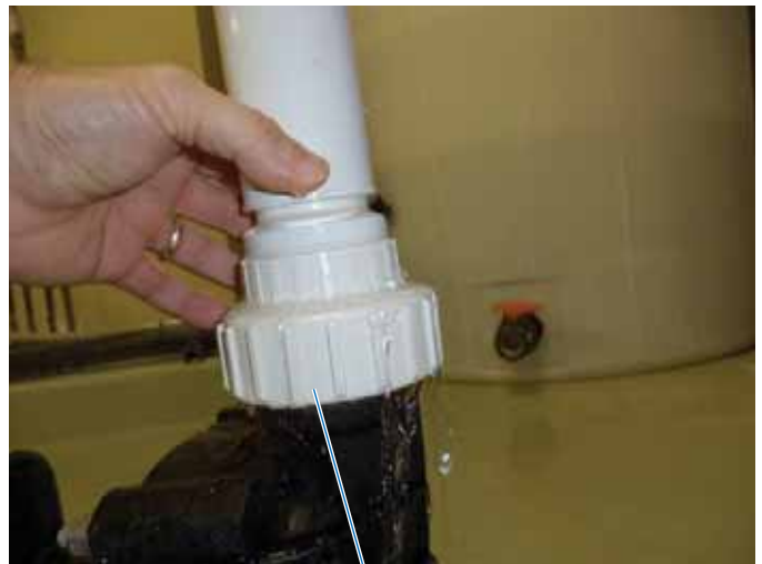
Tighten union after pump is primed with water.
