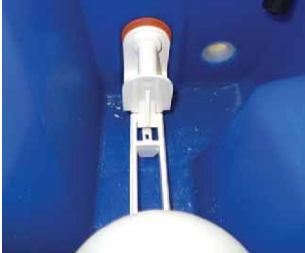
Note position of Gasket inside Feeder Base
